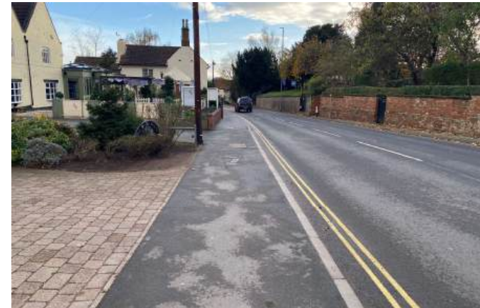
Church Street – there is only a footway on one side of the street, which is relatively narrow, and decreases below 1.5m in width towards the junction with Ollerton/Mansfield Road
