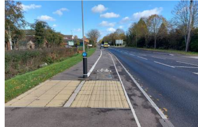
Farndon Road – While there is better separation between people walking and cycling on this section, the cycle track is inadequately wide to provide for cycling in both directions
